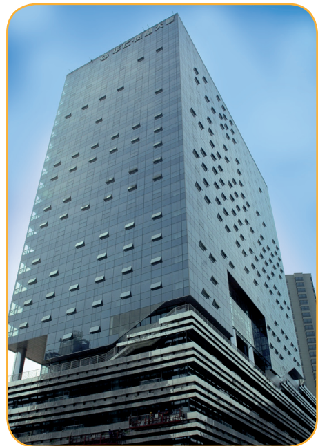
Business building construction Phase 1 „Wuxi“
